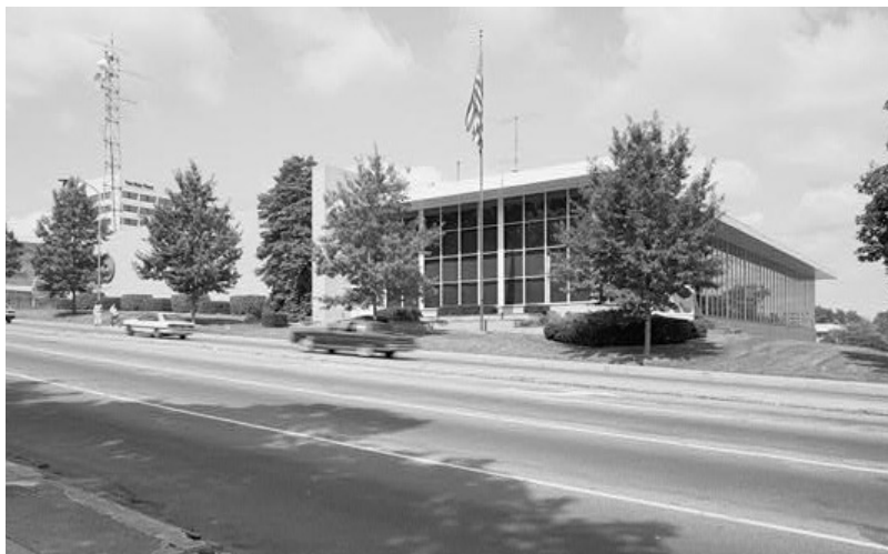
Historic HABS Photograph of WCAU Television Station
